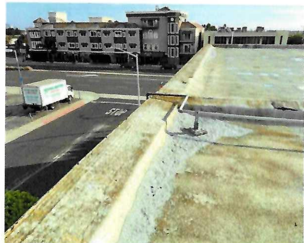
12. Close-up photo of granules collecting in the corners of the roof.
